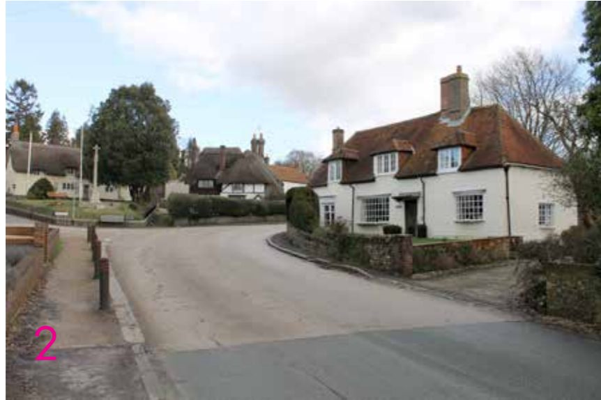
Buildings press up against the street and deflect the road around them, creating spaces off them that lead to lanes and alleys.
