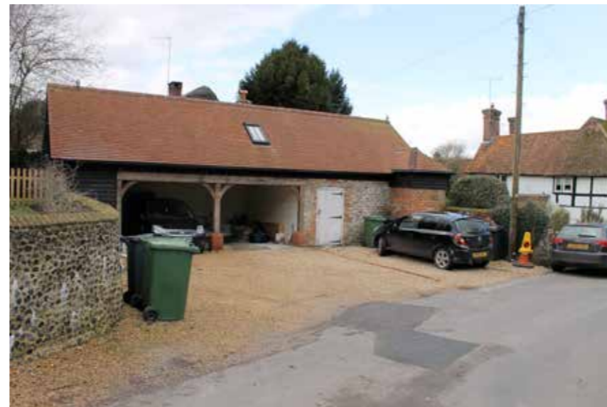
Car parking barn in side road plot with local materials with built in store and roof space use. The use of wheely bins without place to store them does compromise the clarity of the space.
